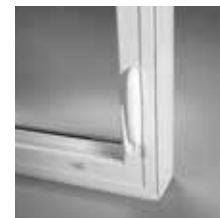
Awning windows feature a dual locking system on each side of the window.
